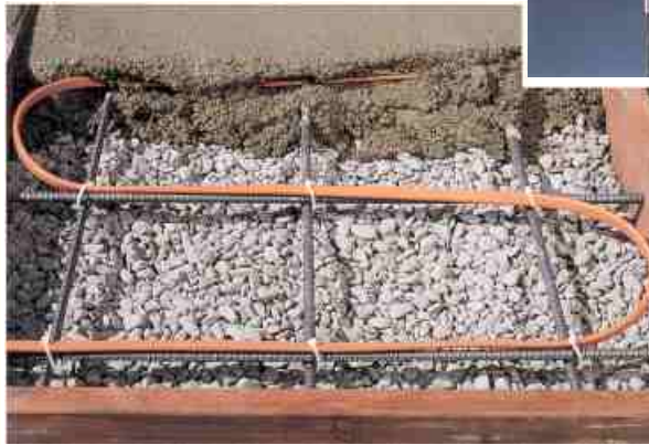
Installation is easy. Simply tie the heating cable to the rebar.....
